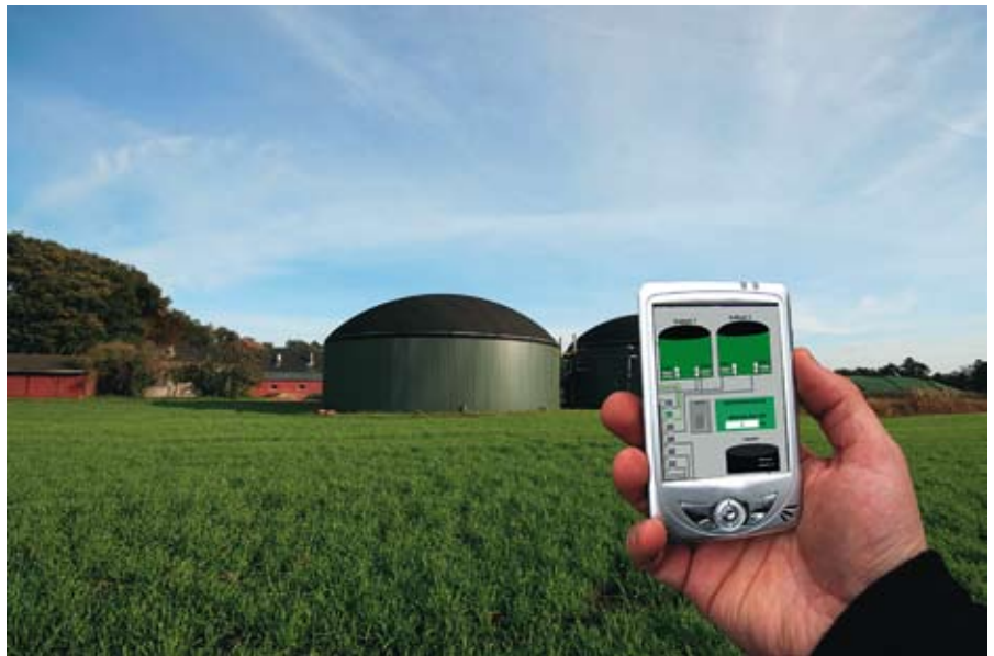
▲ Mobile solutions in the PlanET plant control system ensure that all components of the biogas plant are under control at all times.
